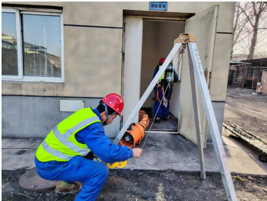
Drilling at limited space
