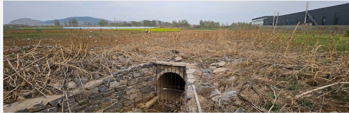
Linyi Farm support the construction of Tanglin Village drainage ditch
