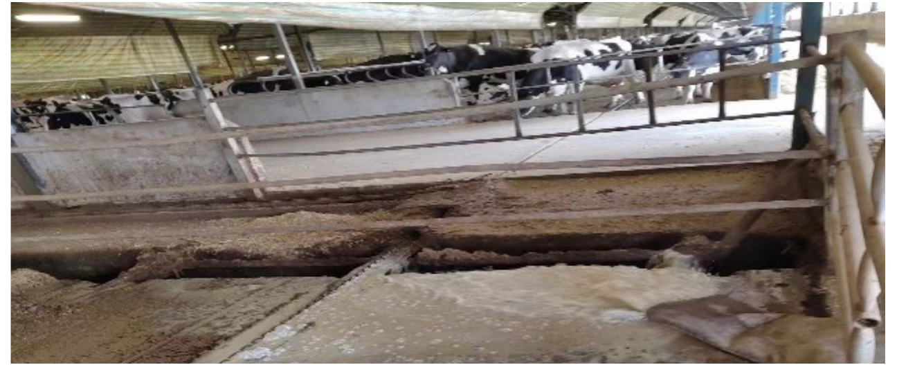
Biogas slurry and manure water used to backwash the cowshed manure channel
